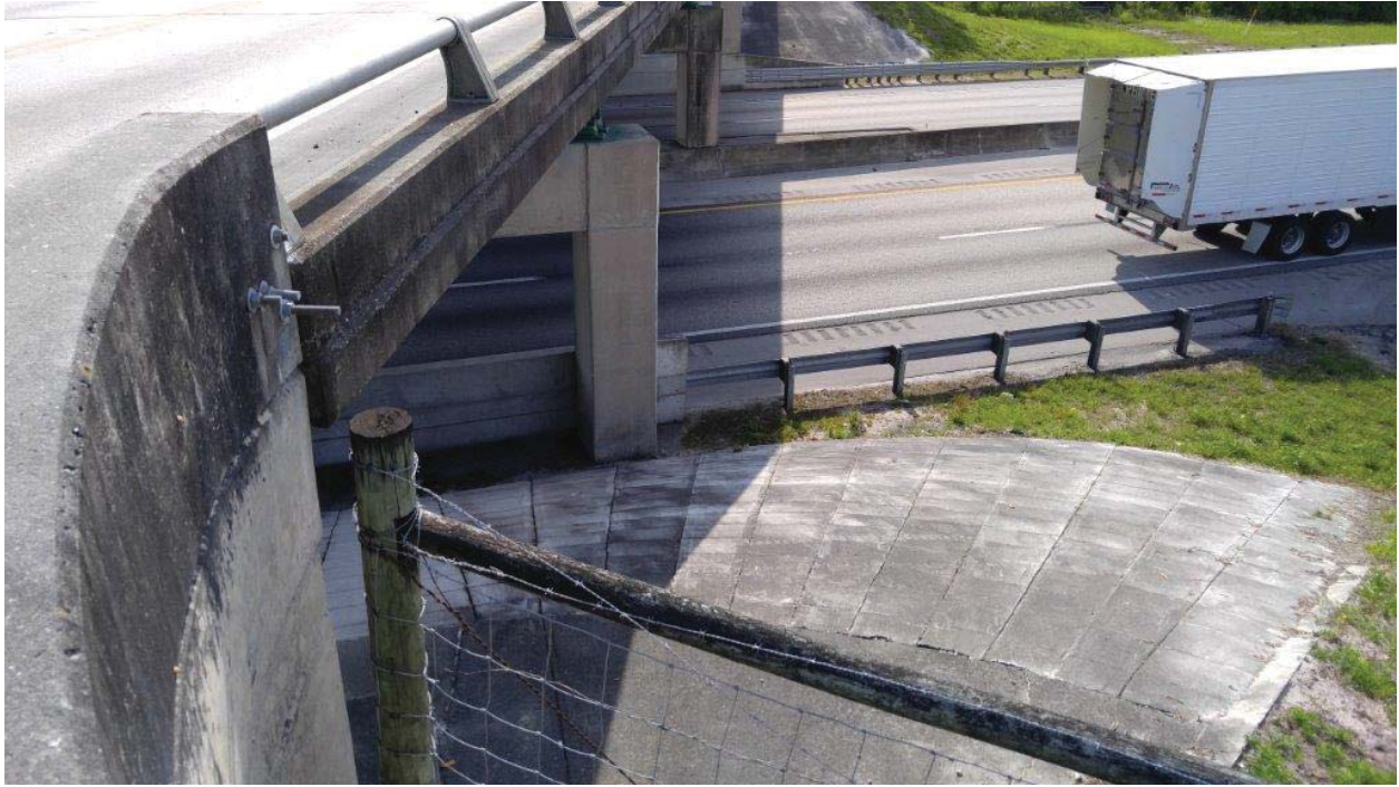
Homogeneous Area #1 White Painted Caulking (samples 1, 2, and 3)
