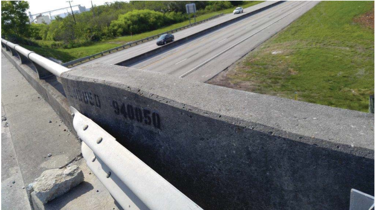
View of FDOT bridge number
