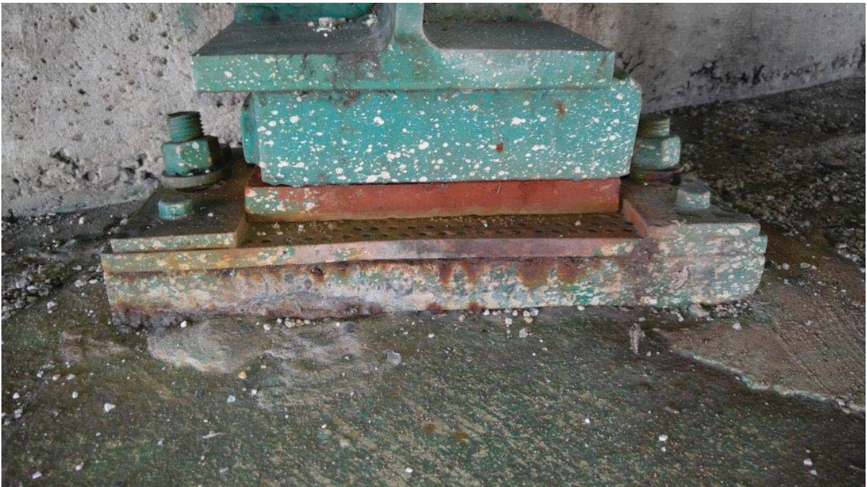
View of bearing pads (all metal)
