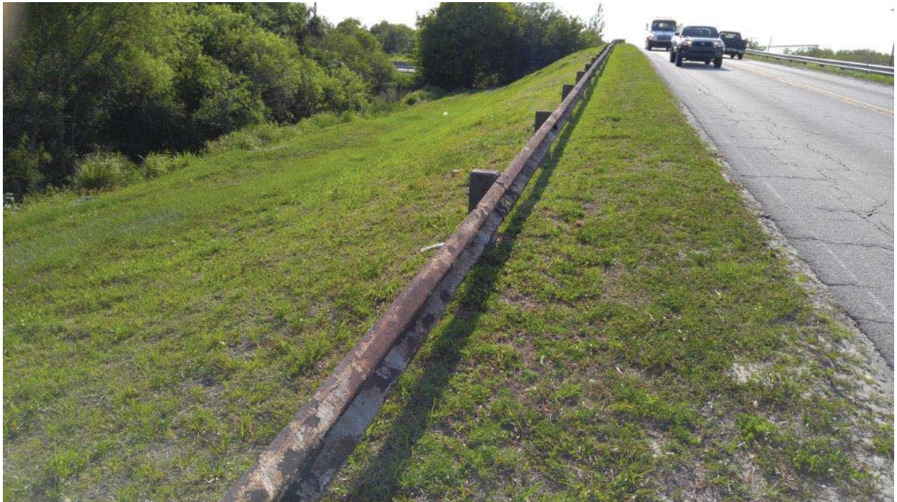
Guardrail South-East (LBP sample #2)
