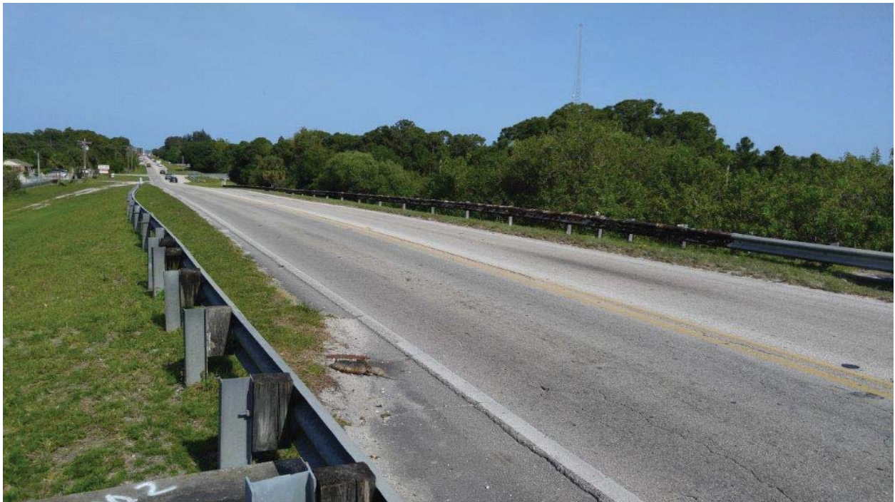
Guardrail near bridge (southeast guardrail) (LPB Sample #4)
