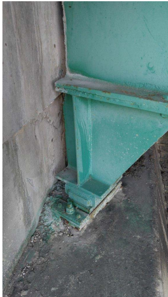
Sample # 7 Concrete – bridge abutment
