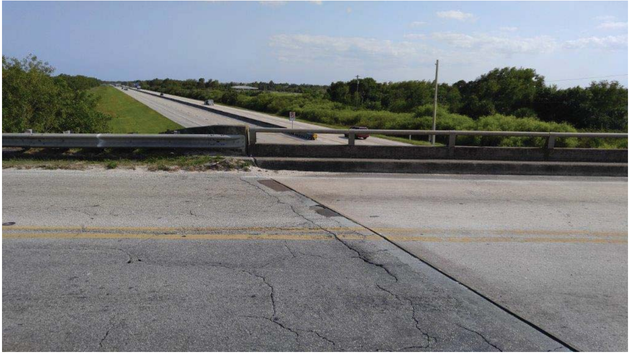
Homogeneous Area 2 – Black joint compound Top Deck (samples 4, 5, and 6)
