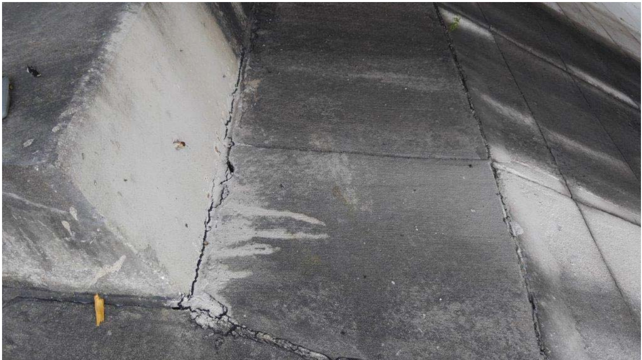
Homogeneous Area 1 – White Painted Caulking retaining wall under deck (samples 1, 2, and 3)
